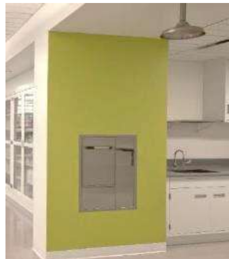
Safety Stations & Eyewash
